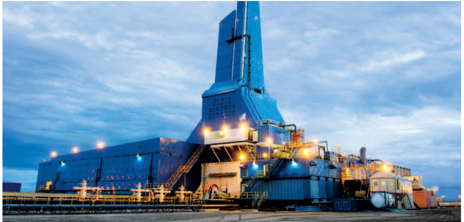
In Sakhalin, Russia, leading-edge technology was applied to drill extended-reach wells from the shoreline to the Chayvo field. This allowed for horizontal drilling under the sea floor and eliminated the need for a second offshore platform while minimizing and in some cases eliminating environmental risks.
