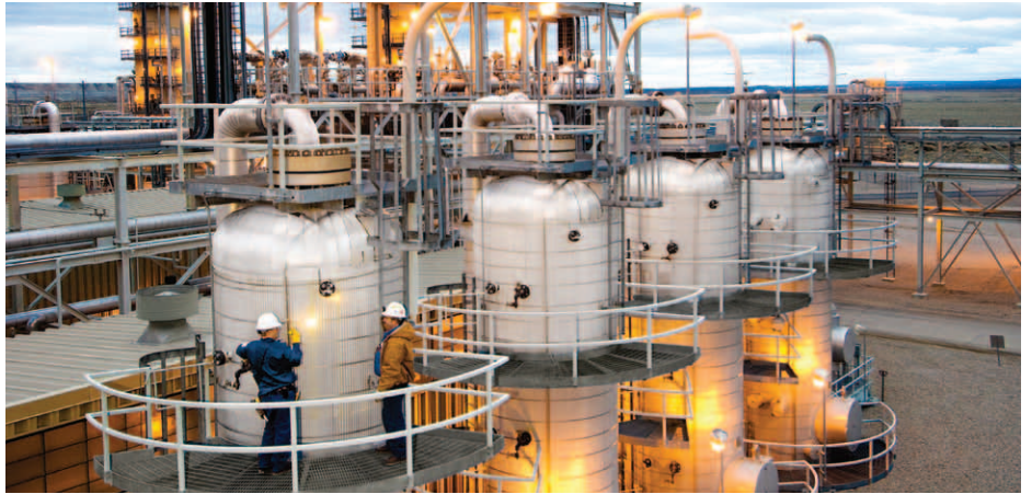
In 2010, ExxonMobil completed an expansion of the world's largest carbon dioxide capture plant located near La Barge, Wyoming. The expanded plant will help reduce GHG emissions and enhance oil production in the United States.
