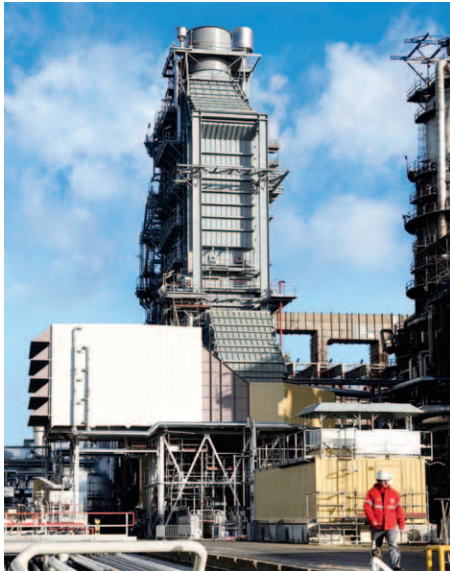
Energy efficiency is one of the most effective tools available for reducing GHG emissions. The high efficiency cogeneration plant at the Antwerp refinery in Belgium reduces Belgium's carbon dioxide emissions by approximately 200,000 metric tons per year.
